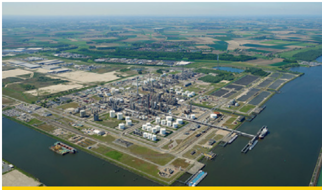
We are taking steps to reduce emissions from our existing operations, including at our Moerdijk petrochemicals complex in the Netherlands, where we invested in new furnaces that reduce energy consumption and emissions.
